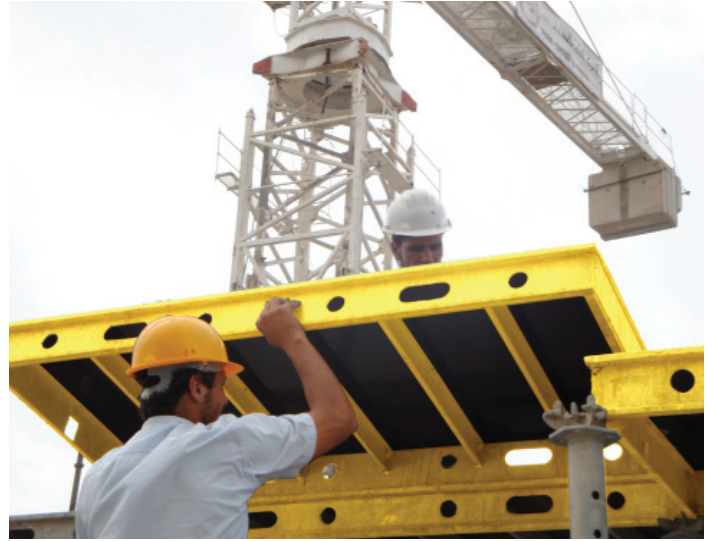
B. Support the panel in the corner using the Top Deck Bearing as illustrated.
