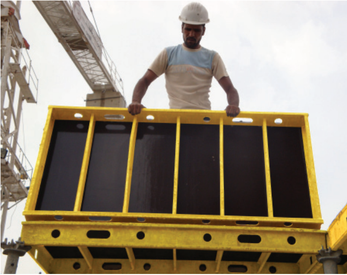
A. Place the Alu Top Deck panels onto the Top Deck Bearing from above.
