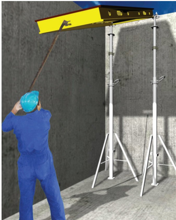
C. Using the Alu Erection Rod, swing up the panel and push it onto the Top Deck Bearing until it is secured properly against the wall.
